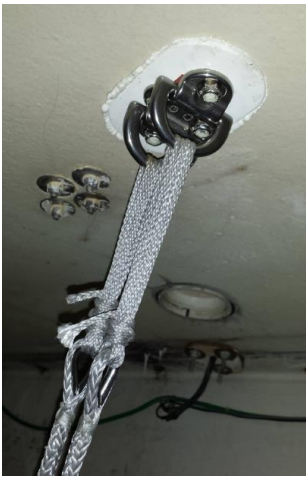
Padeyes under the deck, Spectra lashing.
