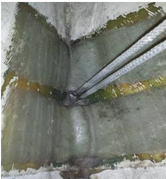
Inner forestay anchor glassed into hull.
